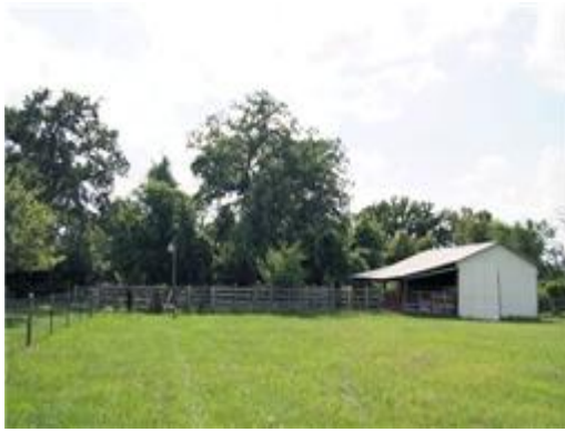
Outbuilding w/ attached pen
